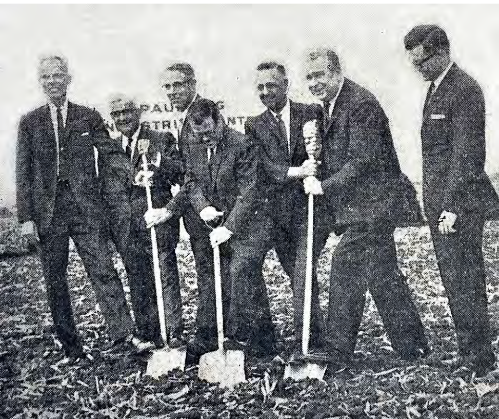
June 1966: Gov. James Rhodes attended groundbreaking ceremonies for an industrial shell building on Road 144 (Gasser Road) in Paulding. From left are Homer Mentzer, president of Paulding County Community Improvement Corp. of Paulding; A.N. Prentice, vice president and general manager of Ohio Power Co.; C.R. Young, local Ohio Power branch manager; Mayor Ab Rife; Don Parker, county commissioner; Gov. Rhodes; and Rev. Hal Zug.
