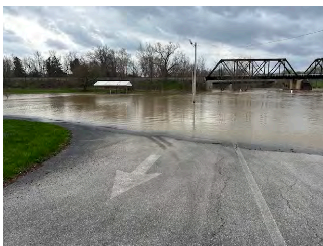
The Park in Oakwood struggles to stay above the flood lines during epic storms like the ones of March 31 st and April 4 th .
