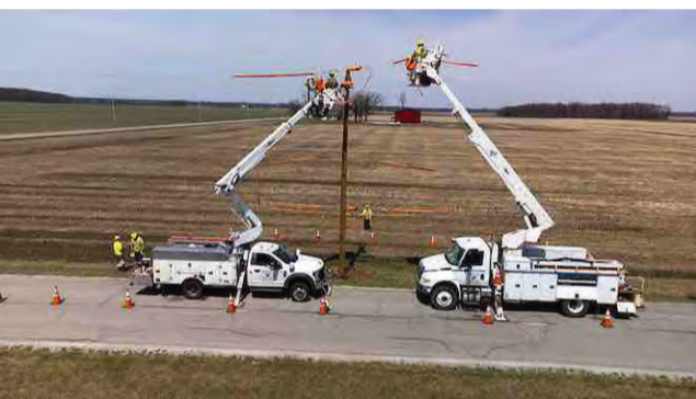
PPEC linemen work on a pole replacement.
