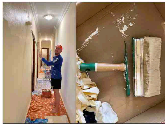
About halfway into the painting project, I had a new, "professional" paint brush split in half.
