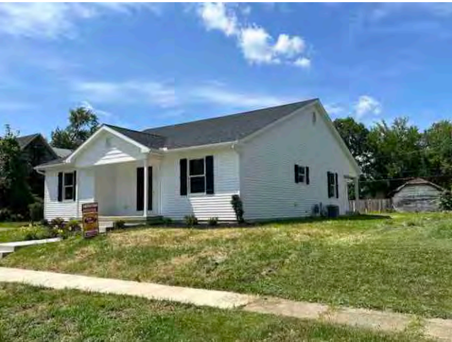
Vantage Carpentry, Electrical, Construction and Equipment Technology students complete construction of this home located at 143. E Raymond St. Van Wert, OH.
