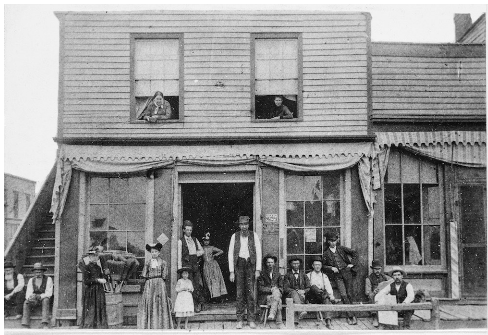
Coon Long - Grocery Cor. Main & Railroad Street
