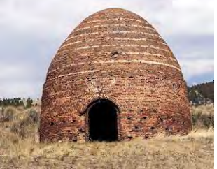
An example of a beehive kiln, similar to ones located in Paulding County in the late 1800s. Paulding Furnace covered theirs with lime plaster, making them "white as snow."
