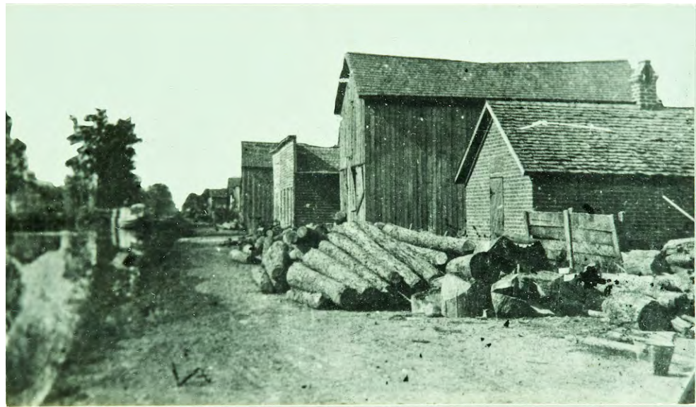
Along the Canal - Looking West from Main St.
