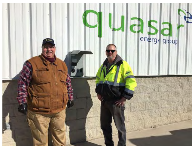
Fred Pieper and Bruce Weidenhamer check out the emergency power panel at the digester at Haviland Drainage Products.
