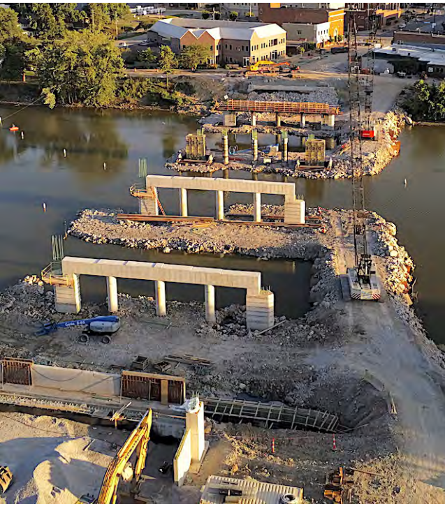
Clinton Street Bridge on August 10, 2019
