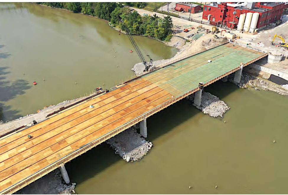
Latest on the Clinton Street Bridge progress - taken on September 21st.
