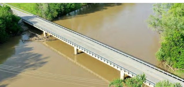
Cecil Bridge at Country Road 105
