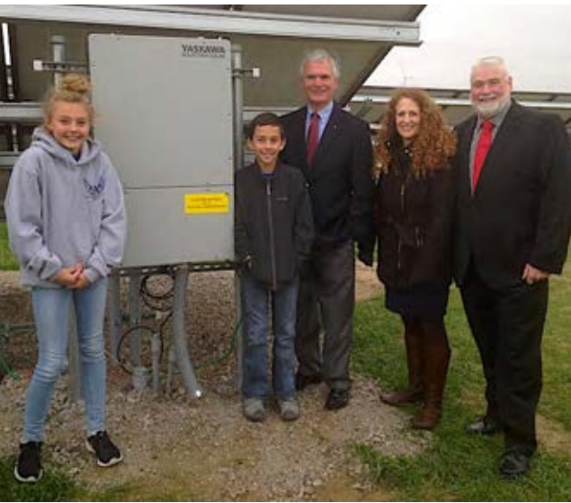
Samantha Sheedy, Aiden Lichty, Representative Bob Latta, State Board of Education - Lynda Haycock, and Antwerp Tech director, Harold Gottke, turn on the power for this massive field array.
