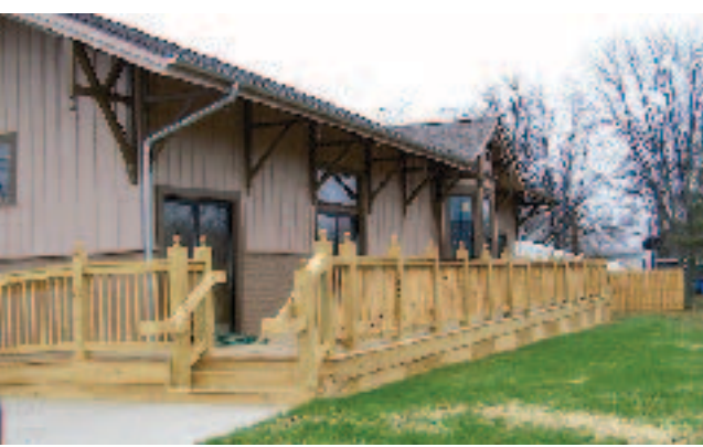
Antwerp's Norfolk & Western Depot built in 1880, recently restored and used by the Village. The video walk-thru and pictures are at www.westbendnews.net
