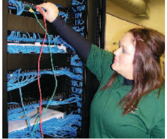
Vantage Network Systems junior, Audrey Smith from Wayne Trace, verifies the connection on the network distribution panel in lab.
