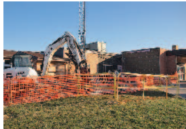
Paulding County Hospital new ER construction
