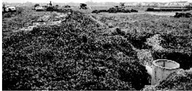
(Breaking Ground Continued from Page 1)
