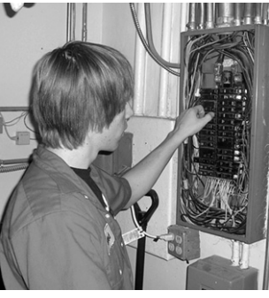
Vantage senior Electricity student Brad Goodwin (Parkway) traces a circuit in a breaker panel while working on a project at the Van Wert YWCA.
