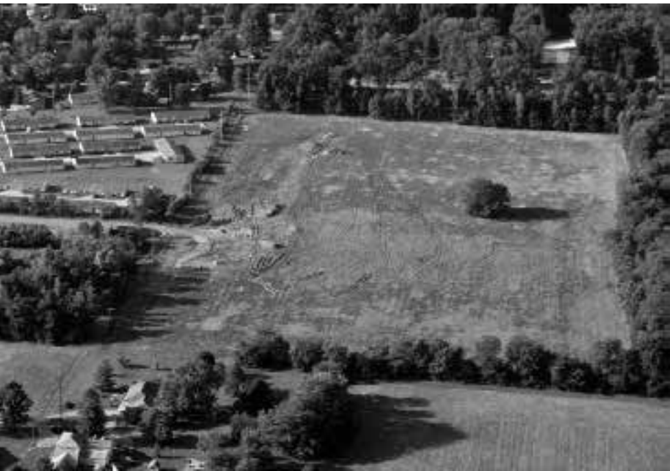
Aerial view of the future "Maumee Landing"
