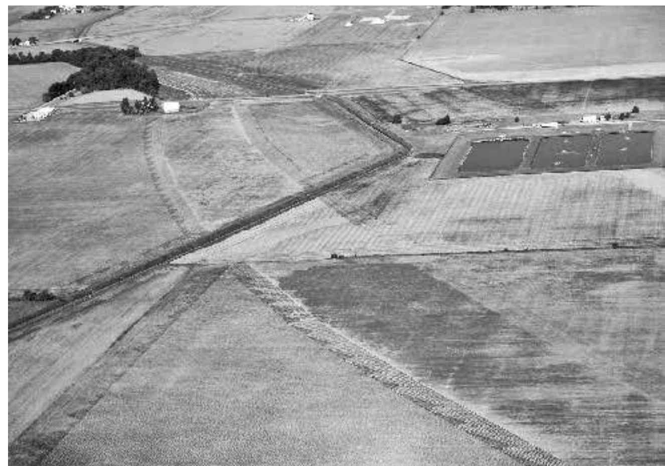
Future US24 seen under construction from aerial shot viewing west.
