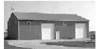
OR348 - Gigantic 48'x72' (3456 sq. ft.) pole barn w/approx. 1564 sq. ft. of living area inside including 3 BR., 1 1/2 ba., family & living rooms. The remaining workshop has (2) 12'x14' overhead doors & 16' ceilings. Pond & 6.4 acres of land. $129,900.
