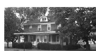
OR373 - 5-6 BR, 2-story brick home on 2.3 acres with out-buildings on S.R. 111, Paulding. $99,500
