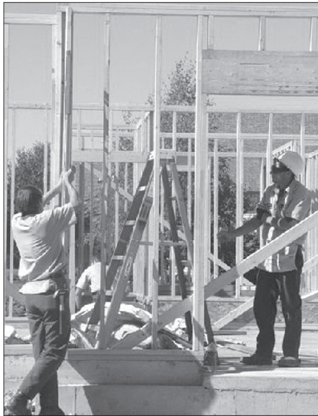
Vantage senior carpentry students work on framing this year's construction project
